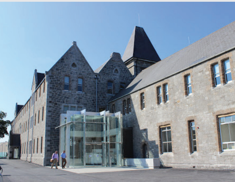
The North House was built in 1854 and was designed by Murray & Denny. The building was refurbished in 2014 as an academic space for TU Dublin. It will be further developed as part of the University's Academic Hub & Library due for completion in 2023.
